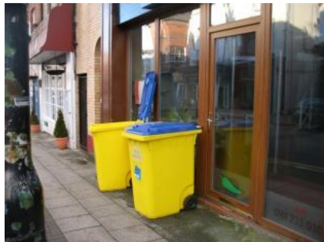
Photograph 23: Modern Shop Front
