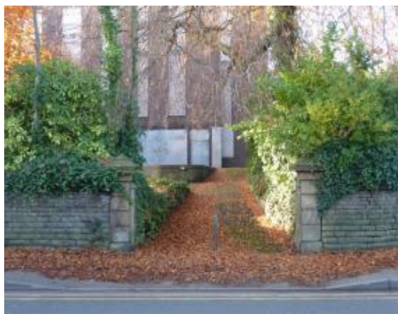
Photograph 35: YWCA, Ashley Road
