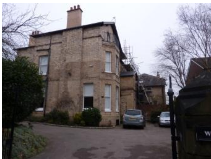
Photograph 38: Loss of Garden
