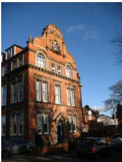
Photograph 52: Telephone Exchange, Woodville Road
