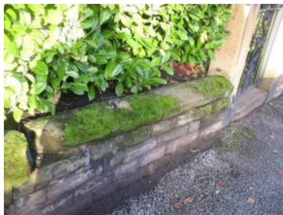
Photograph 13: Stone Wall with Evidence of Railings
