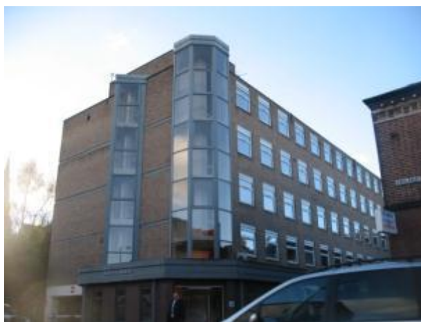
Photograph 19: Ashley House on Ashley Road
