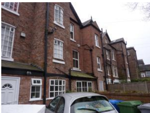
Photograph 36: Rear of Osborne Terrace, 17-23 Hale Road
