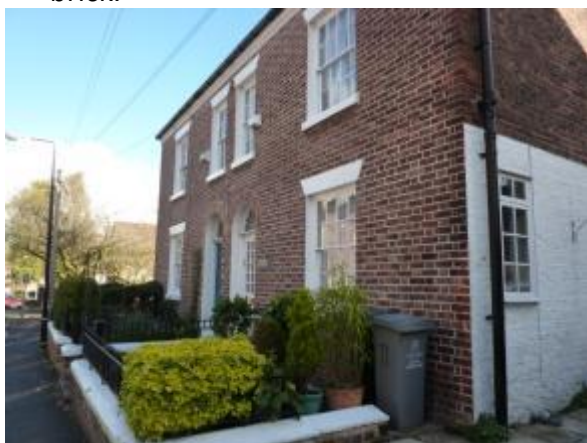
Photograph 12: Town Garden with Boundary Wall and Railing
