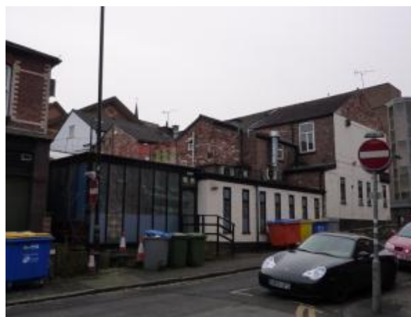
Photograph 37: Rear of 19-23 Ashley Road
