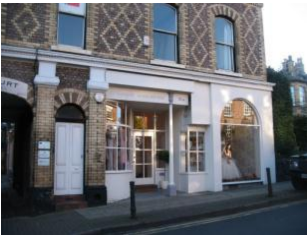
Photograph 22: Modern Shop Front Incorporating Pillar, with Brick Detailing Above
