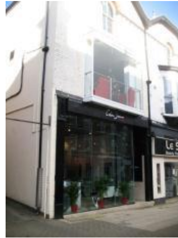
Photograph 41: Inappropriate First Floor Window
