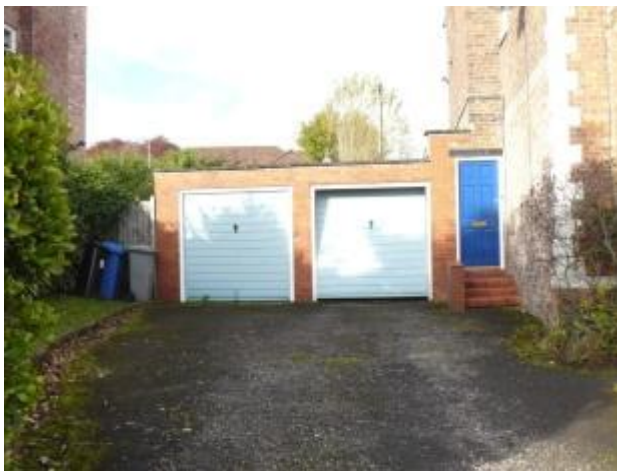
Photograph 42: Intrusive Garage/Hard Standing on Lyme Grove (Wide Opening not Visible)
